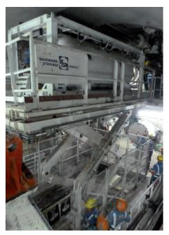
Figure 2 : TUP shuttle being mated to TBM lock
