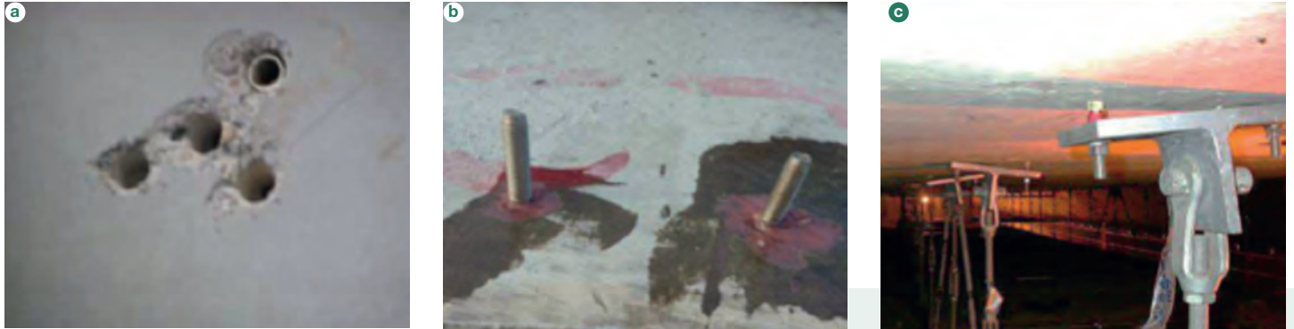
Figure 51 : Issues with post-installed anchors: a) drilling, b) installation quality, c) fixing failure
