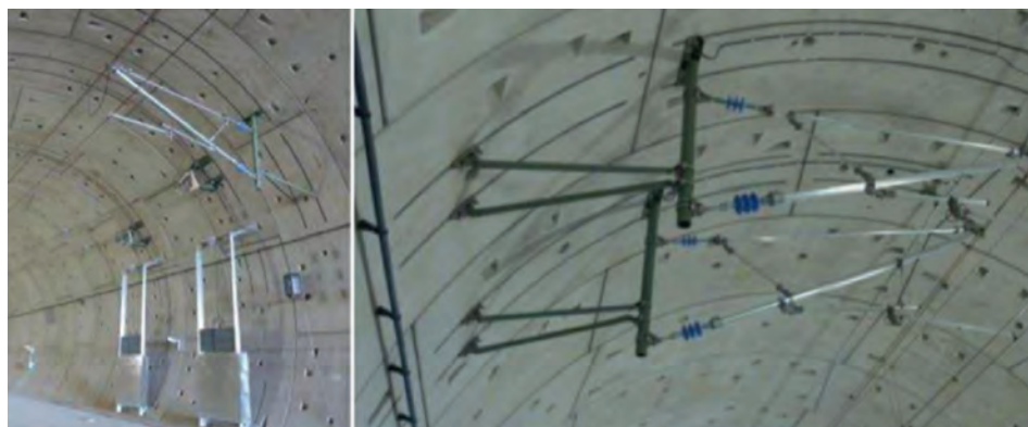
Figure 54 : Curved cast-in channels used as fastening system in railway and high-speed rail tunnels
